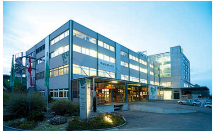
Robatech Headquarters - Muri, Switzerland
