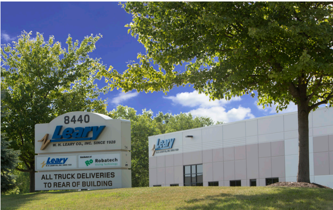
Leary Headquarters - Tinley Park, Illinois, USA
