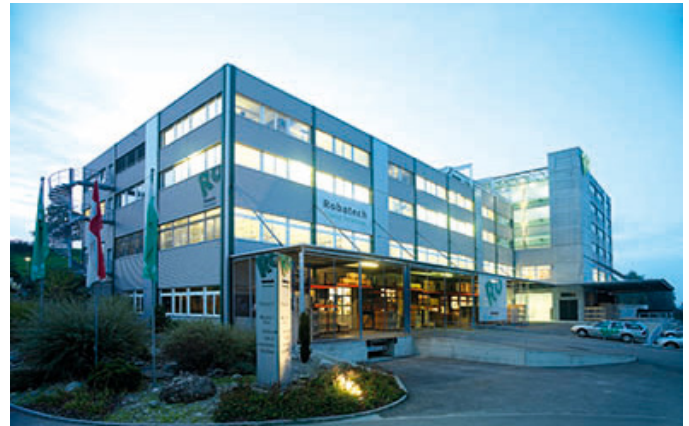
Robatech Headquarters - Muri, Switzerland
